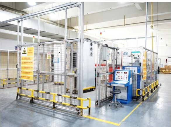
Voltage Withstand Test of Switchgear
