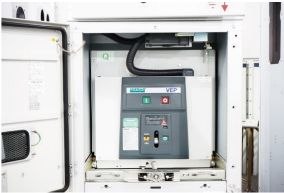
Circuit breaker in service position
